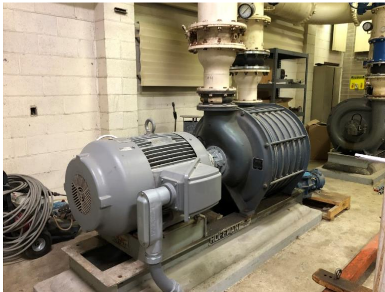
Figure 1. SAM's existing 125-hp Aeration Blower
