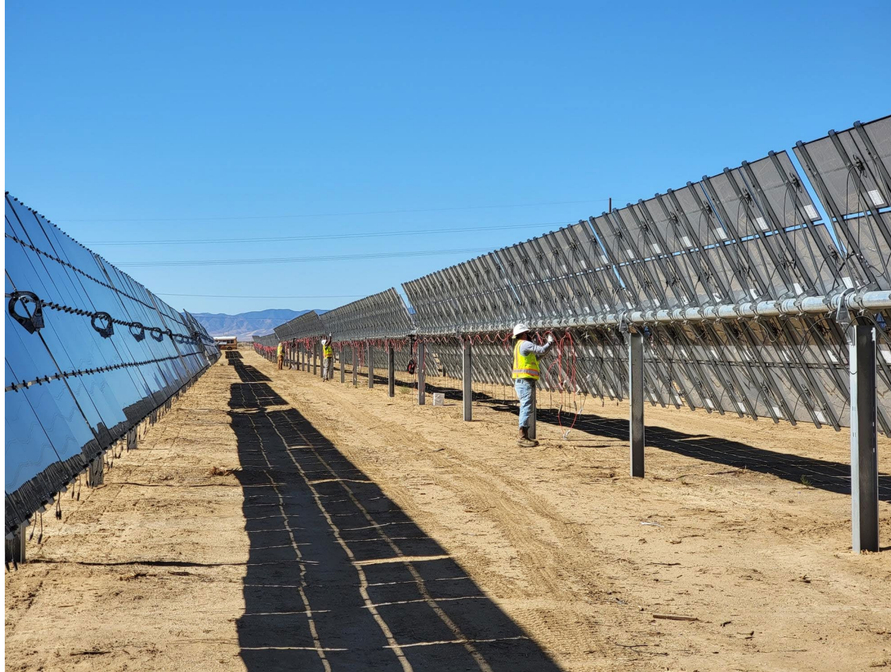
Courtesy of Leeward Renewable Energy (Chaparral Project) – Installing wire harness
