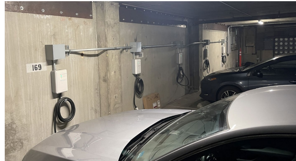
Power-Managed Level 2 Chargers
